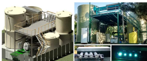
Fig 1. Multistage treatment strategy for urban leachate remediation along with the main results (up) and scheme/photographs of the full-scale plant (bottom).
